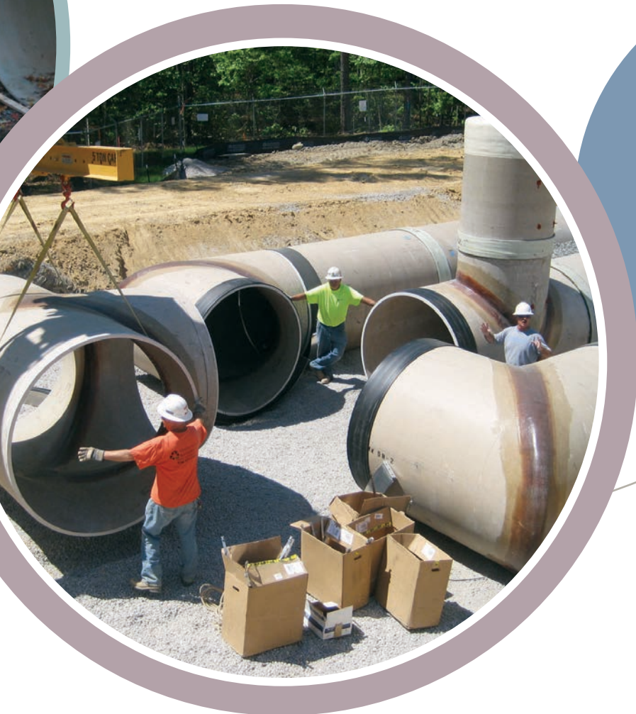
The custom fittings and intake structure manufactured for a slipline installation at a coal-fired electric power generating plant included this 110 by 84-inch reducer. (Above) Custom made elbows and tees create manifolds for an underground containment reservoir. (Left)
