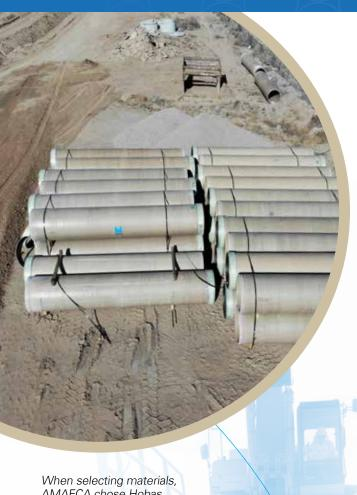
AMAFCA chose Hobas centrifugally-cast, glass-fiber-reinforced, polymer mortar 42-inch and 36-inch pipes with tee bases and 30" flanged tops to serve as irrigation piping for agriculture.
