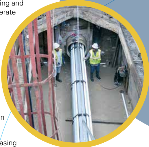
Workers installed the 30-inch carrier pipe by jacking methods.
