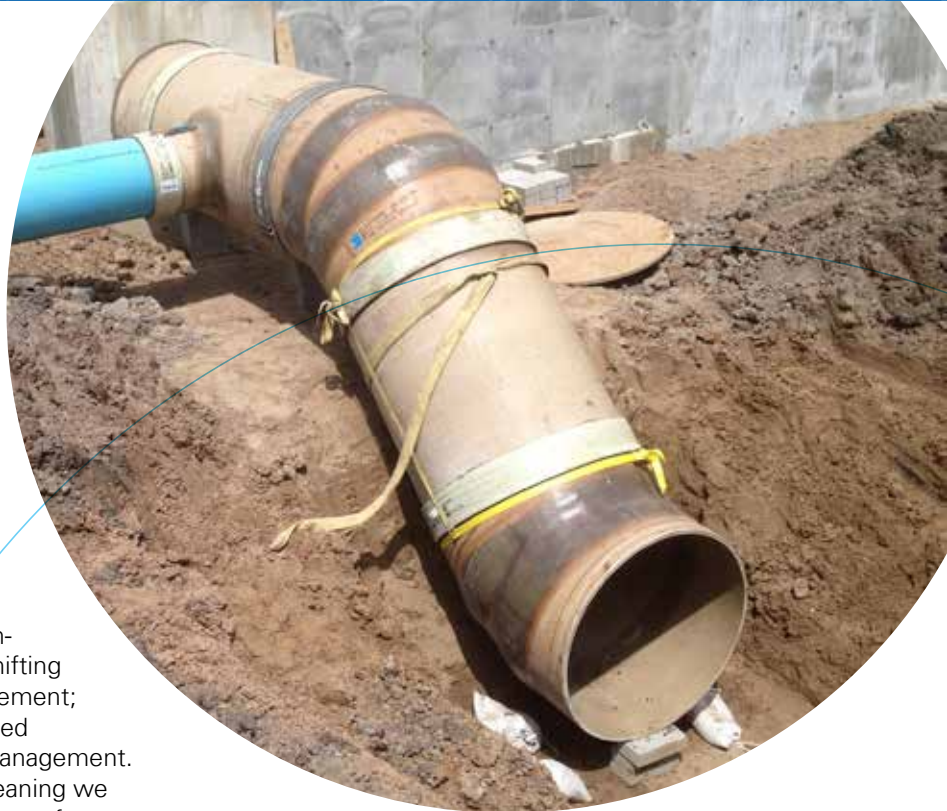
Fittings can be manufactured of the same corrosion resistant material as CCFRPM pipe.
