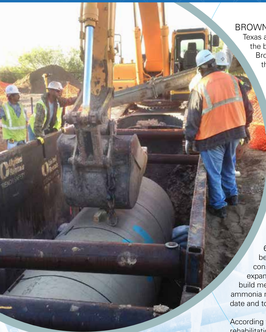
54- and 72-inch CCFRPM pipe was installed by direct bury.
